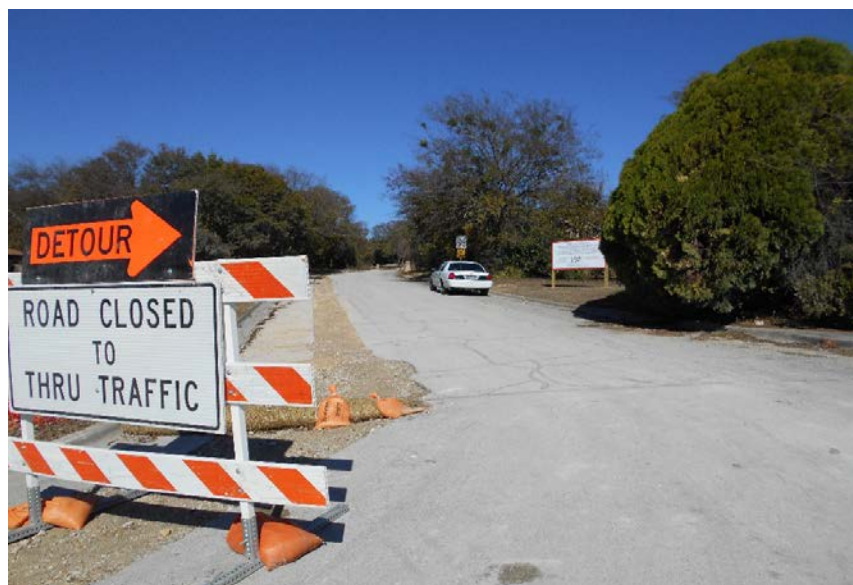
A picture of Rattlesnake Road, where work is to take place.
