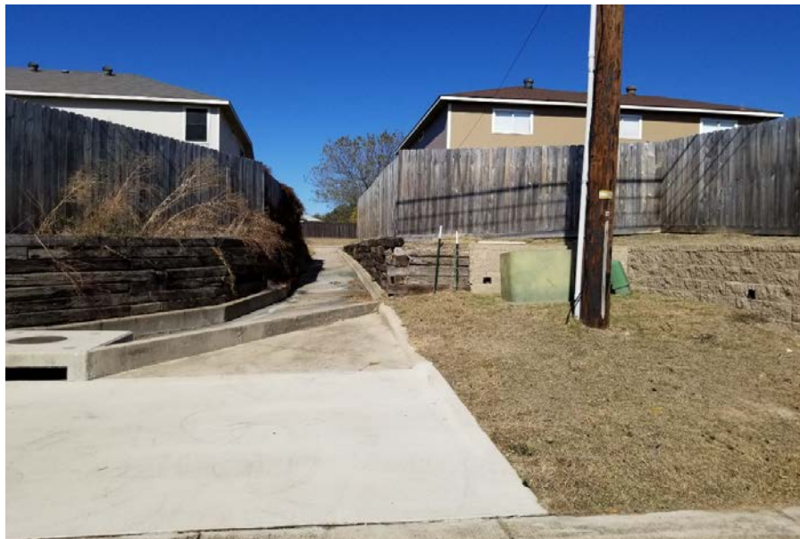
Site of the Drainage Flume Reconstruction Project.
