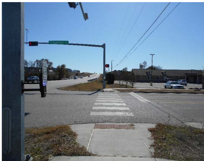
Area of construction for the sidewalk.
